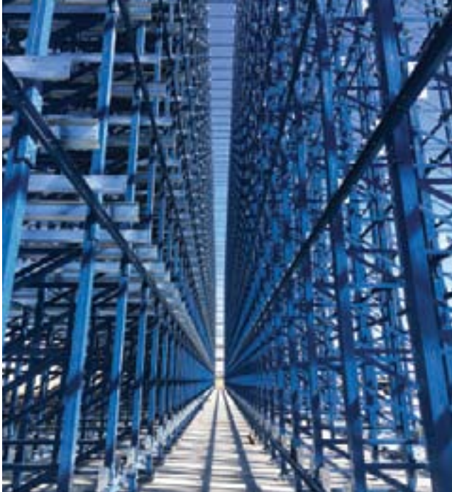
The view down an aisle of the Richland warehouse.
